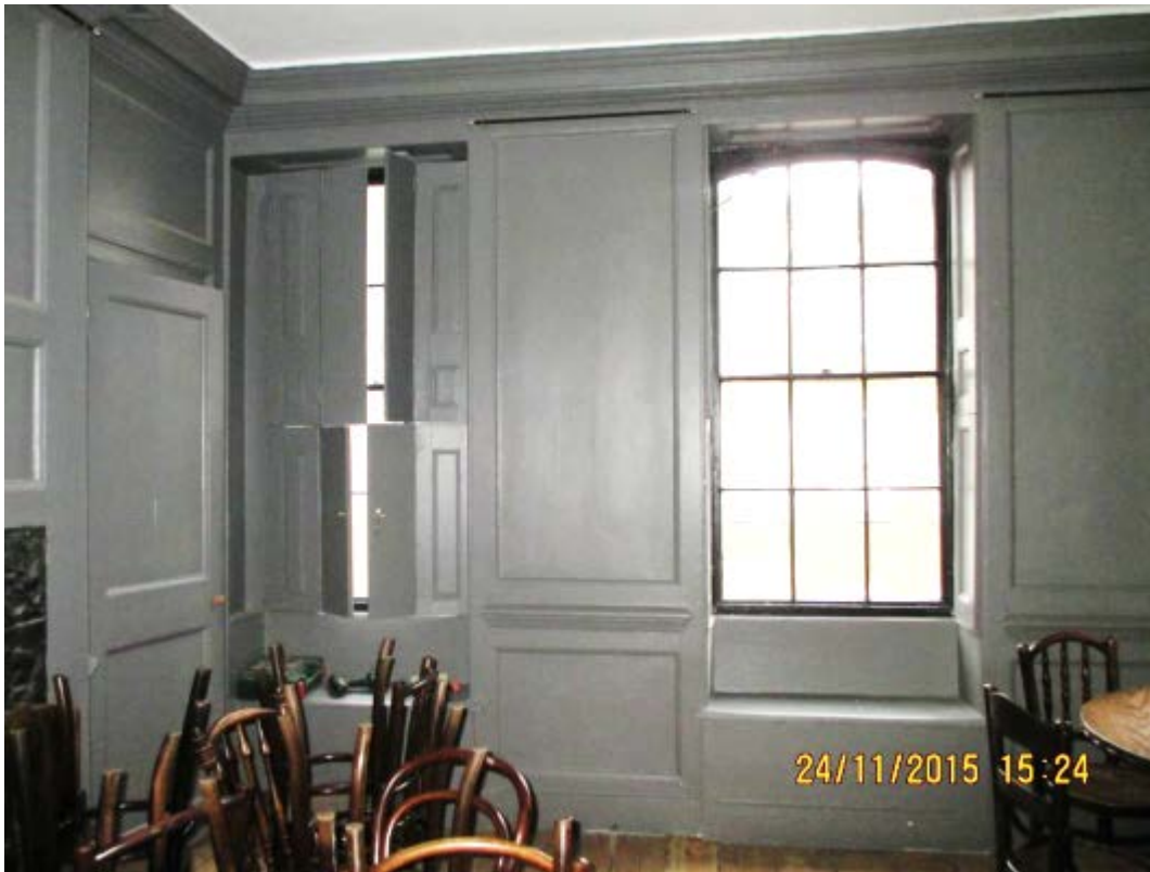
Front room at second floor level
