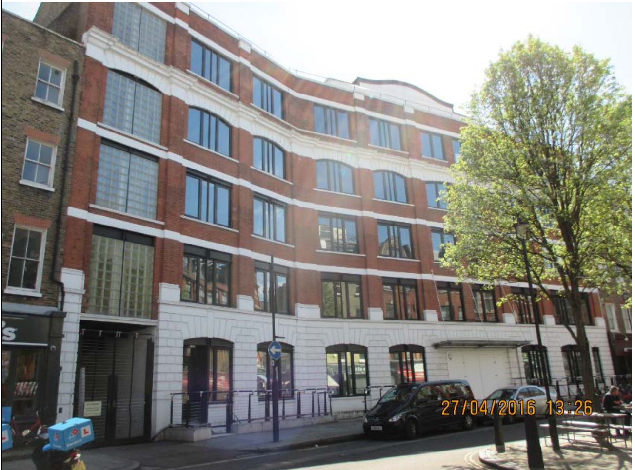
Front elevation of application site facing Foley Street.
